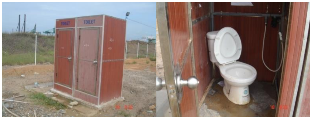
Figure 4.1 Toilets on construction site
