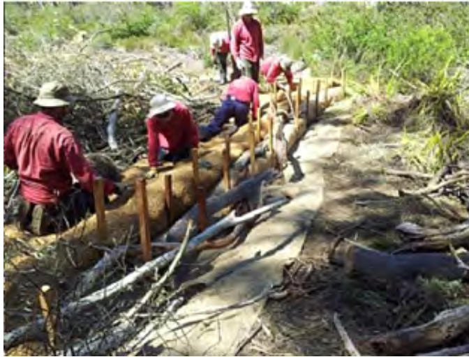
Photograph 2.9: (2014) East Wolgan Swamp Rehabilitation – Water Level Spreader / Retainer Structures
