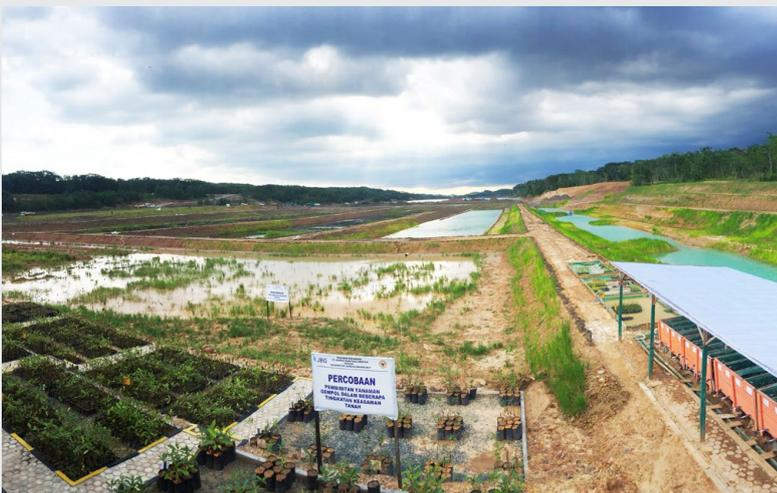
The Company's acid mine drainage management plan covers all mines which have Potential Acid Forming material (PAF). One of the management plans is to improve water quality by chemical treatment such as limestone. For cost-effectiveness, the Company with Brawijaya University conducted research on applying biological treatment for acid mine drainage management. In this research, native plants having the potential to absorb
